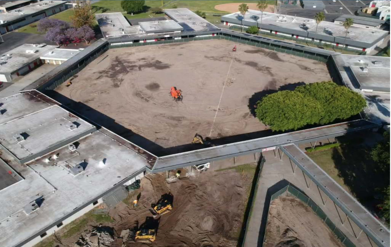
Prepping for the placement of site plumbing.
